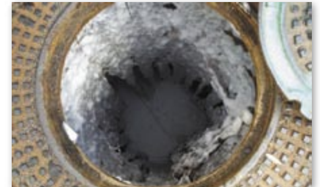
THE ROOT VEIL TREATED WITH VAPOROOTER
